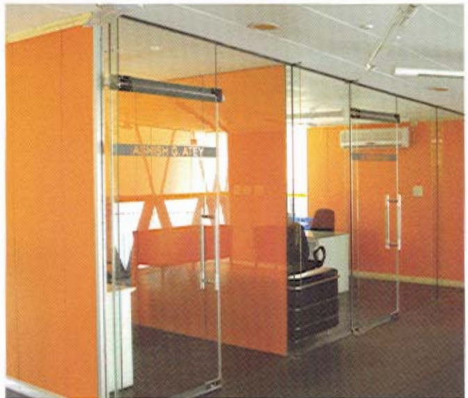
Office - Internal Full Height Wall
