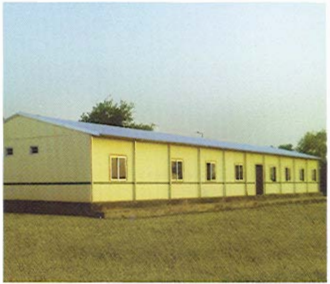
Site Office - External and Internal Wall
