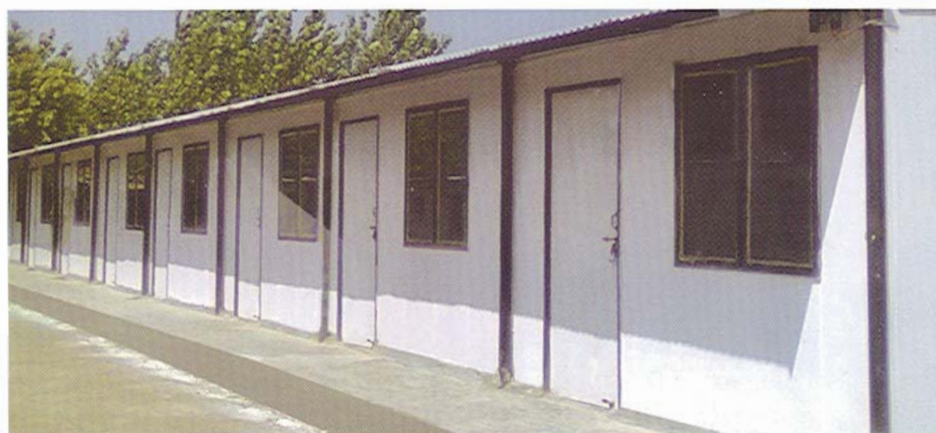
Labour Quarters - External and Internal Wall
